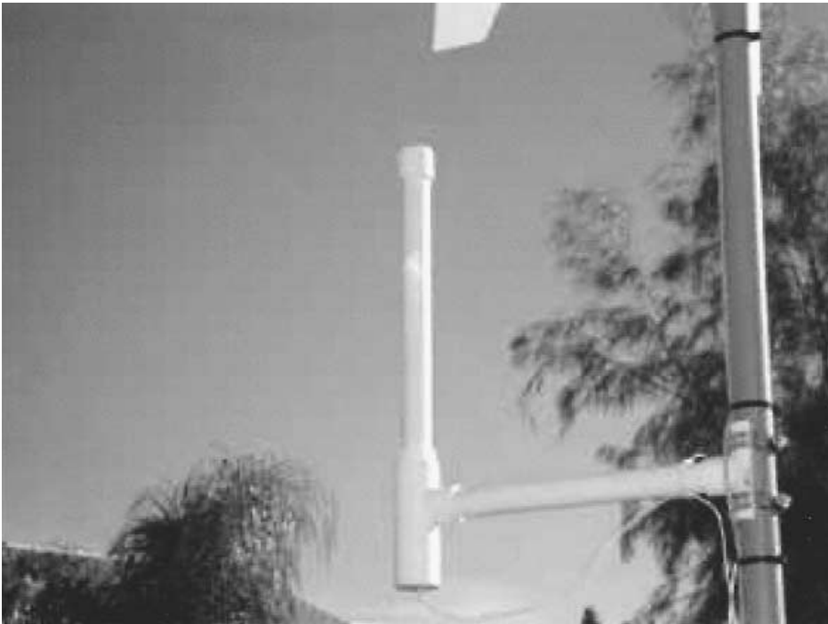
Figure 7-1 Lightning activity monitor.
